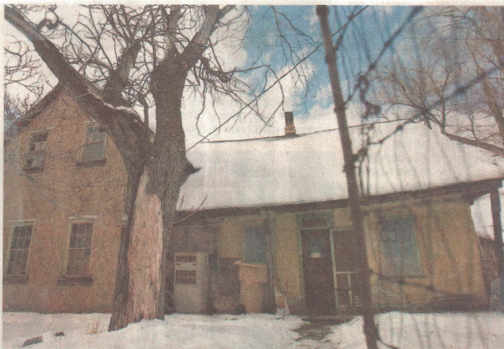
The Levan home of Klarence Meldrum has been condemned, it has no running water and its only heat source is one of two electric portable heaters that keep the house at 60 to 65 degrees.
